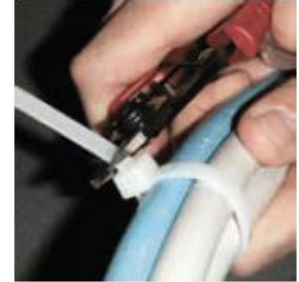
Cut the exceeding part of the tie with the tool, leaving a few mm length as safety.
