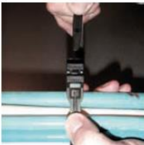
Insert the tip of the tie and tighten a short segment.
